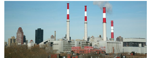
Ravenswood Generating Station, a 2,480-MW fossil fuel plant in New York City
